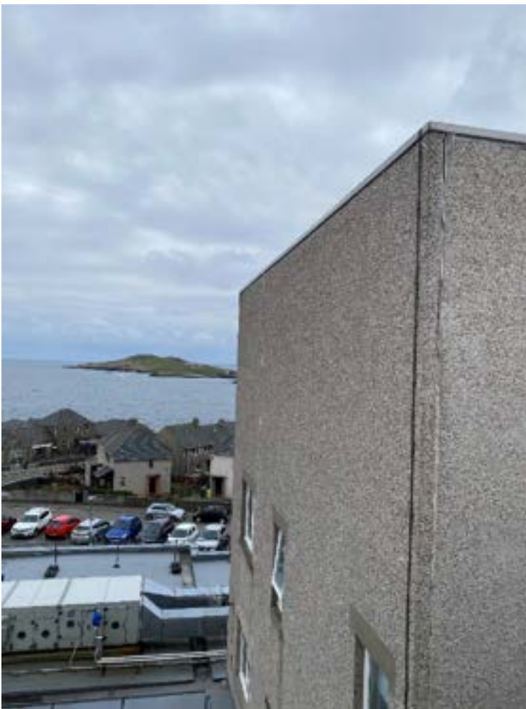
Figure 2.1: View of the east elevation wall from the north
