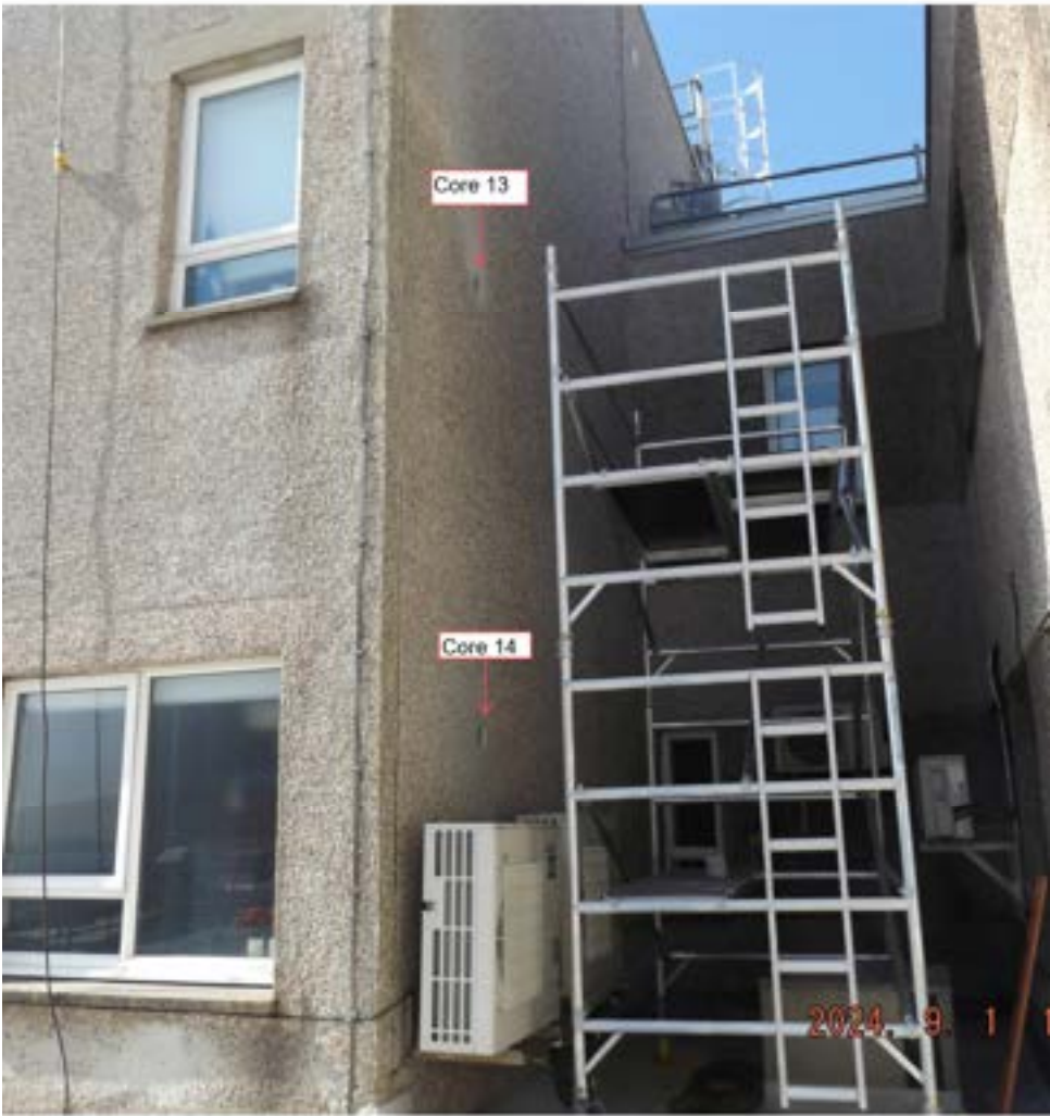
4 Storey North Elevation Wall
