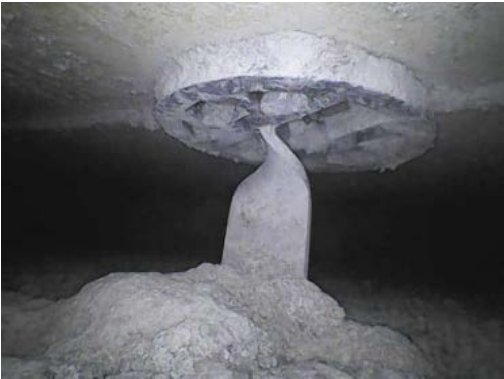
Wall tie at Core 12
