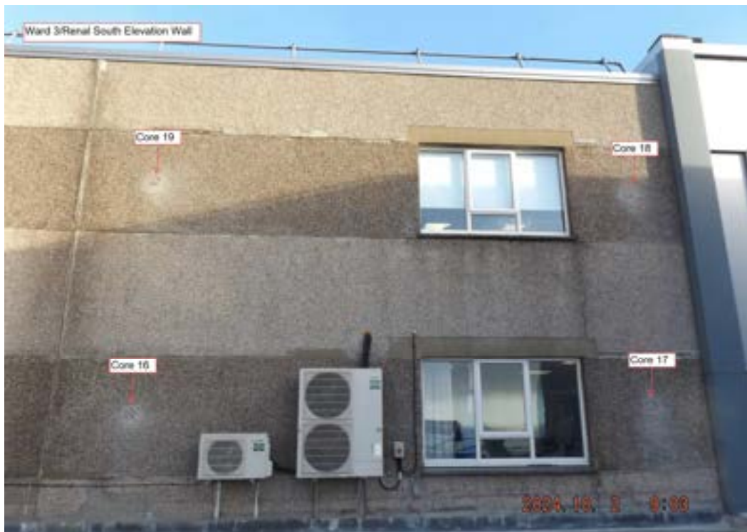
Figure 2.15: Cores at the south elevation of Ward 3 and Renal 2 of 2
