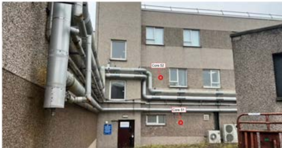
3 Storey North Elevation Wall
