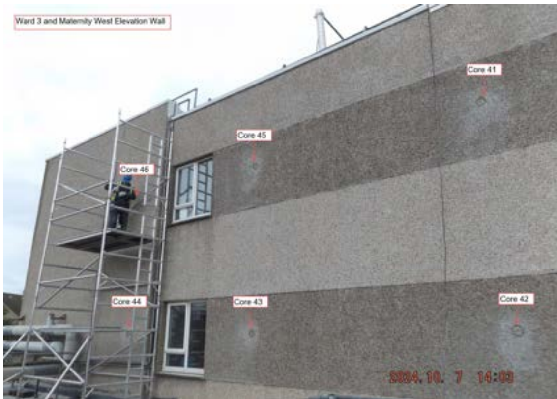
Figure 2.20: Cores at the west elevation of Ward 3 and Maternity
