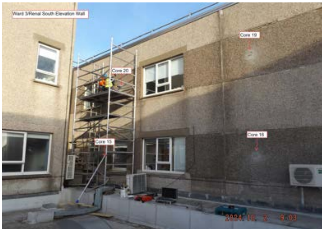
Figure 2.14: Cores at the south elevation of Ward 3 and Renal 1 of 2
