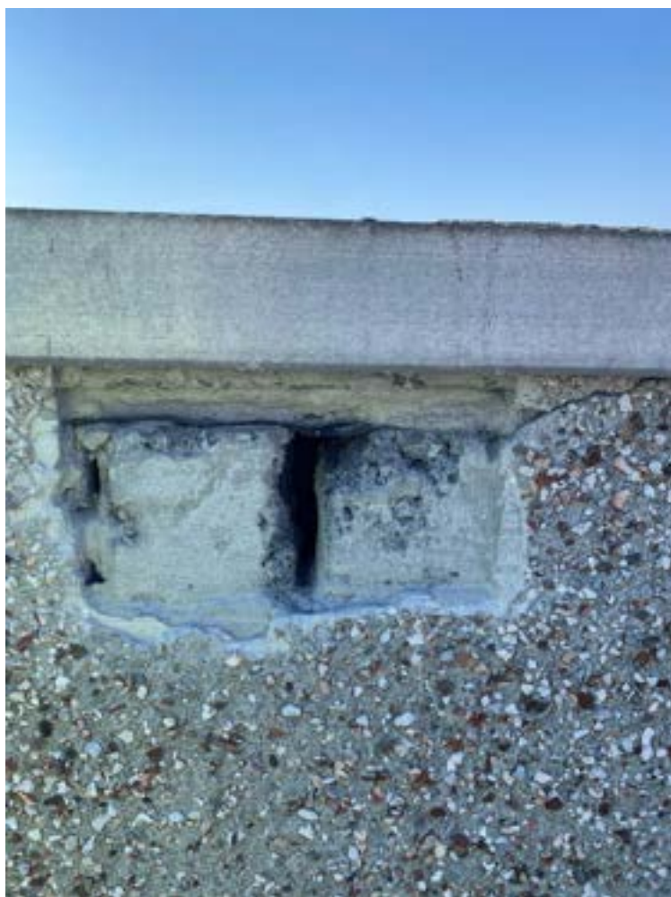
Figure 2.3: Construction at the coping
