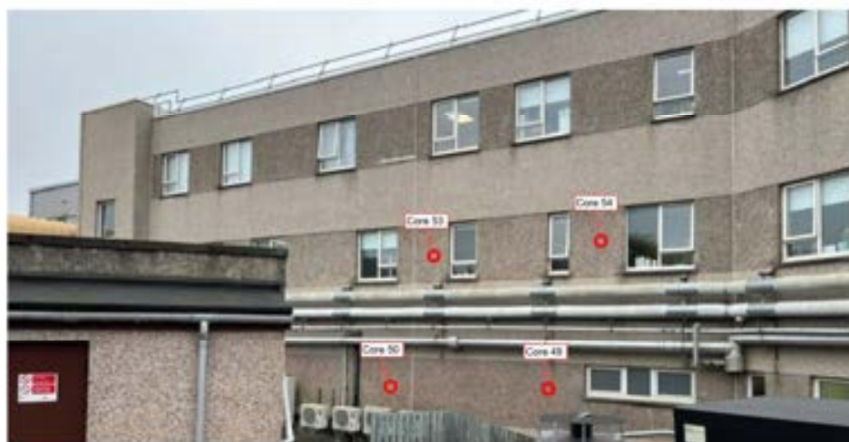
3 Storey North Elevation Wall
