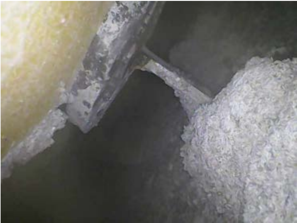
Wall tie at Core 42
