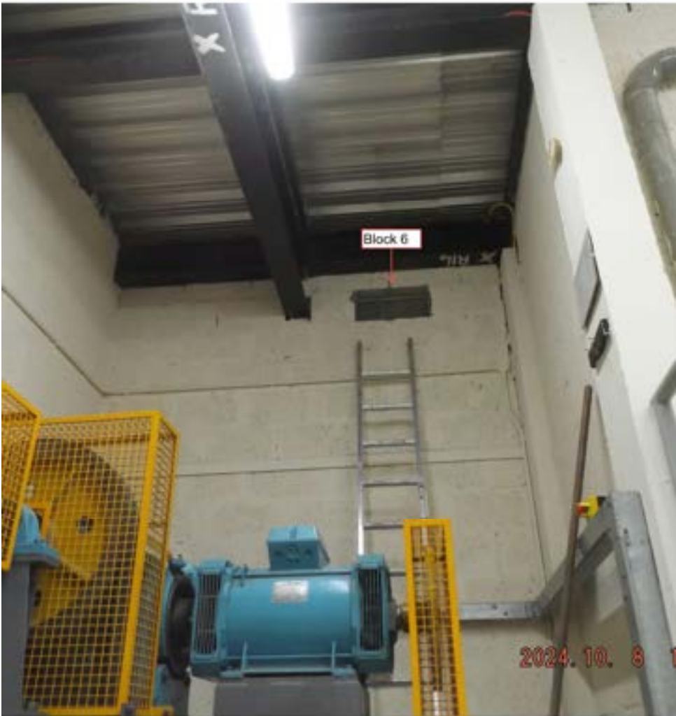
Lift Motor Room south wall
