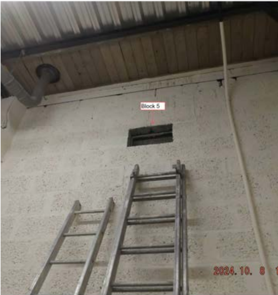
Lift Motor Room west wall
