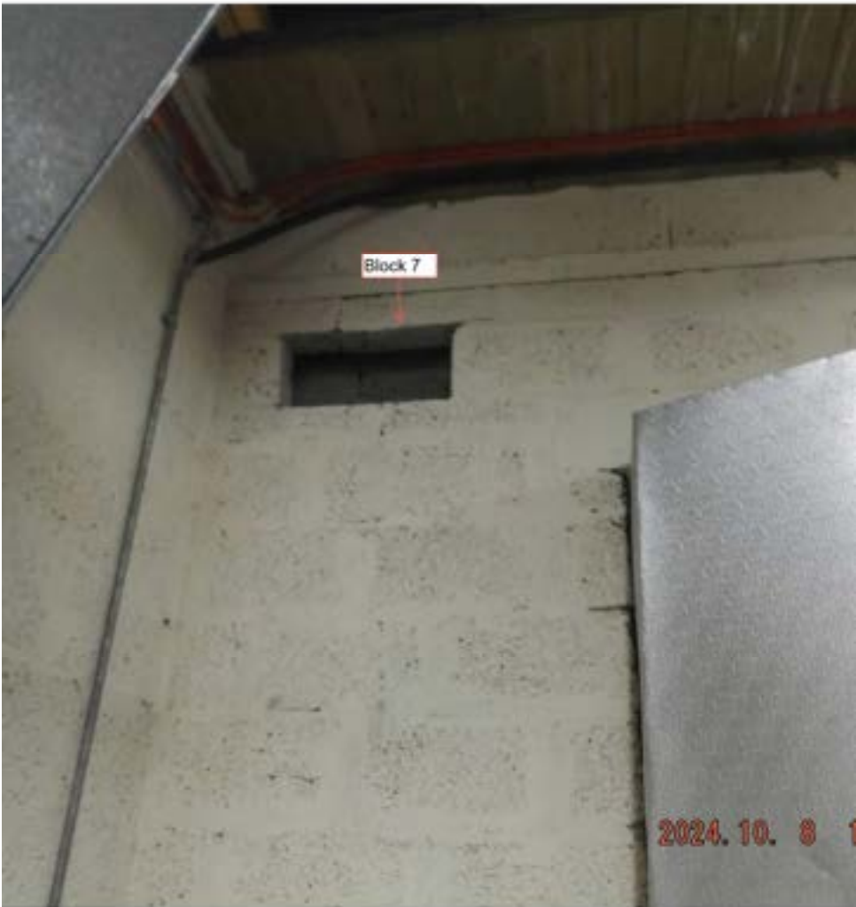
Plant Room west wall
